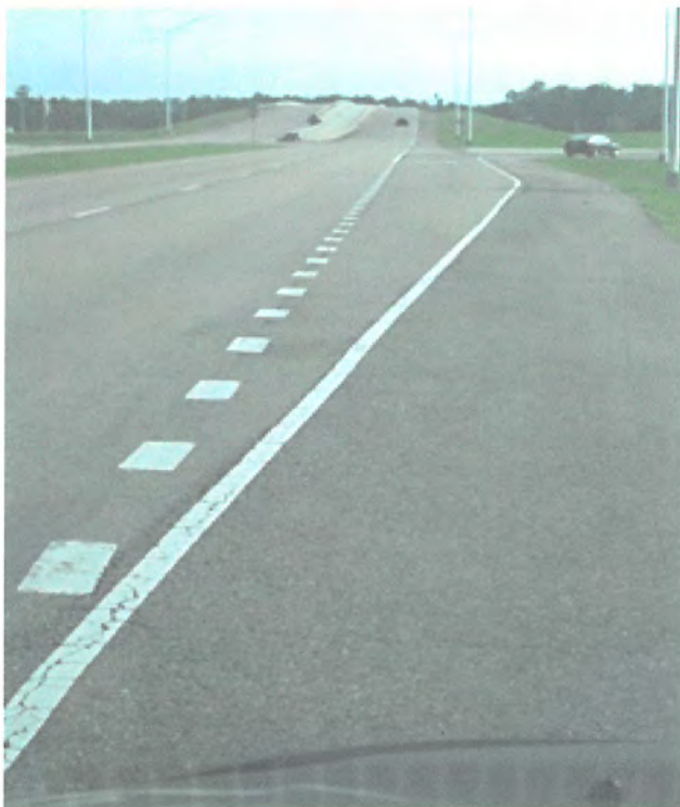
Figure 3: Approaching the I-12 eastbound on-ramp
