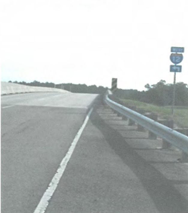
Figure 4: Overpass Shoulder Disappears
