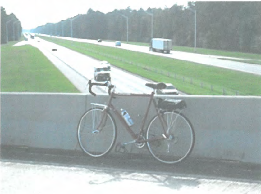
Figure 6: 1088 I-12 Overpass Retaining Wall
